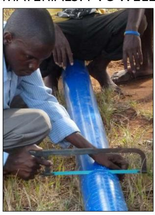
2. For a potable water well for use by a single household or a few households equipped with a rope pump or other low-cost hand pump, a deeper hole may be needed (to protect water quality, so preferably drilled to a second aquifer). In this case a self-slotted 4-inch PVC pipe can be used. In doing so, the well stays relatively affordable.
